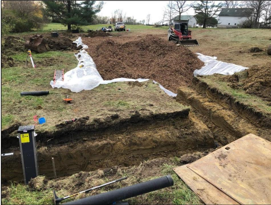
A denitrifying bioreactor is a structure containing a carbon source, usually woodchips, installed to reduce the concentration of nitrate nitrogen in subsurface agricultural drainage flow via enhanced denitrification. One standard 15 ft by 100 ft by 6 ft deep bioreactor system can treat up to 50 ac. If the treatment area at a location was greater than 50 ac, then it was assumed two standard bioreactors would be needed. Locations were identified by an analysis of watershed soils and tile extent.
