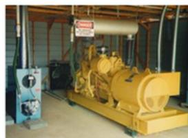
Photo of a 120 kW engine generator set combusts recovered biogas, generating electricity for on-farm use
